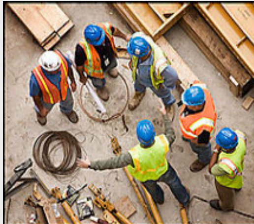
Photo 1: Jobsite Meeting to Discuss Test Protocol
